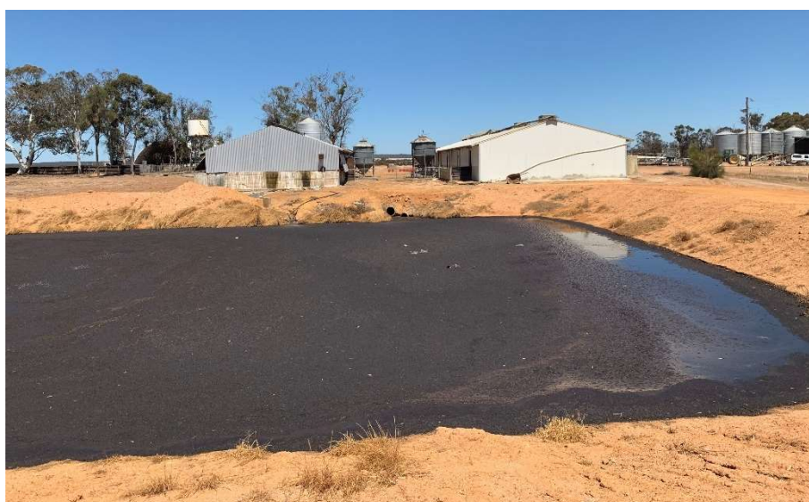
Photograph 4 – Anaerobic Pond
